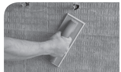
Apply SimpleMat then flatten air bubbles and creases.
