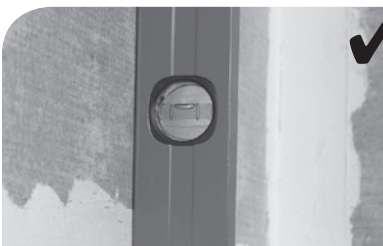
Ensure a flat counter or wall surface.
