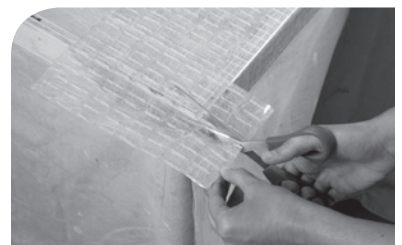
Cut corner from end of mat to facilitate folding of corner.
