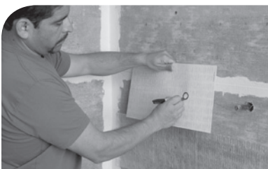
Place SimpleMat in position and mark cuts if needed.
