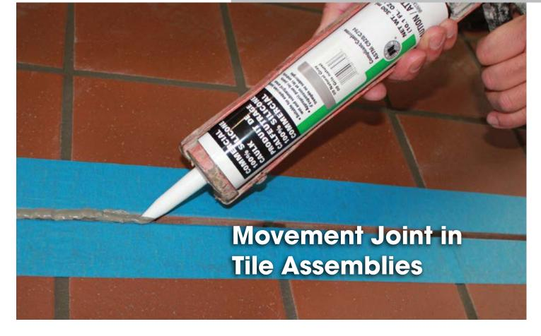
There has been considerable discussion concerning the need for movement joints in tile assemblies. The question is not whether they are needed; that is a simple yes. The questions are "Where do they go?", and "What is used to fill the joint in the tile assembly that will control or compensate for movement in the entire assembly?" There are several different types of construction movement joints defined by the Tile Council of North America (TCNA) that are needed in tile assemblies:
