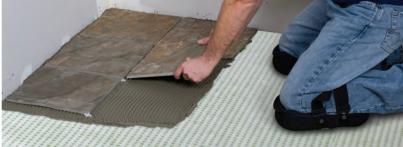
SpiderWeb II is designed differently than bonded membranes. A layer of fabric is bonded to the bottom of the mat to create an air space that helps channel moisture from the substrate below. The plastic and fabric construction will absorb stress created from movement in the substrate and preserve the integrity of the tile installation. The fleece on the surface of SpiderWeb II locks the mortar into the mat, ensuring strong, reliable installation.
