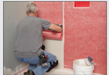
Apply RedGard® Fabric Membrane to walls and floors
