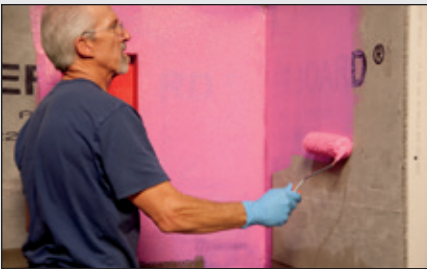
A RedGard® Liquid Waterproofing Membrane over cement backerboard
