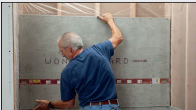
C Plastic sheeting and cement backerboard (for Shower Base only)
