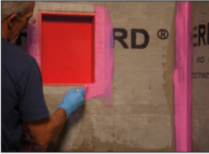
Precoat corners and seams with RedGard® liquid waterproofing membrane
