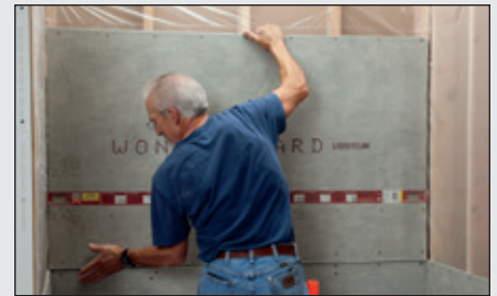
C Plastic sheeting and cement backerboard (for Shower Base only)
