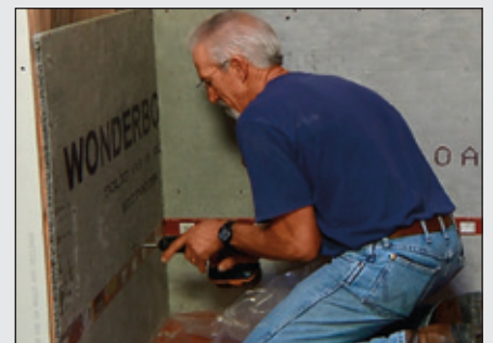
Secure backerboard
