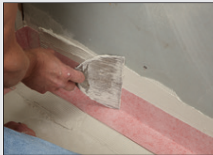
Install RedGard® Fabric Membrane strips for changes of plane
