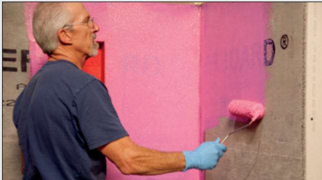
A RedGuard® Liquid Waterproofing Membrane over cement backerboard
