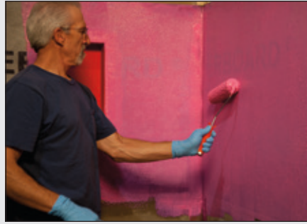
Apply RedGard® to wall surfaces
