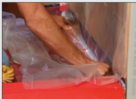
Push plastic into sealant along perimeter
