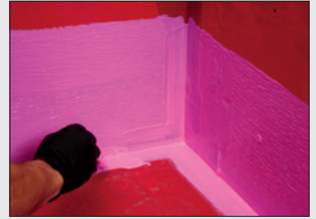
Treat corners and changes of plane with RedGard®
