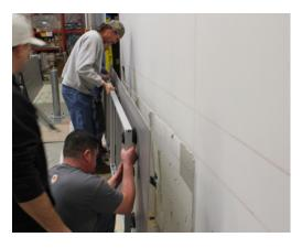
Initially, the thin porcelain tile manufacturers recommended their use on interior and exterior walls only. Now, some manufacturers are also offering tiles that are suitable for interior floor applications. The products recommended for floors are generally thicker and may also be reinforced with a resin-bonded mesh fabric on the back that increases the breaking strength. Professionals should contact the tile manufacturer for the service rating of their tile before installation on floors.
